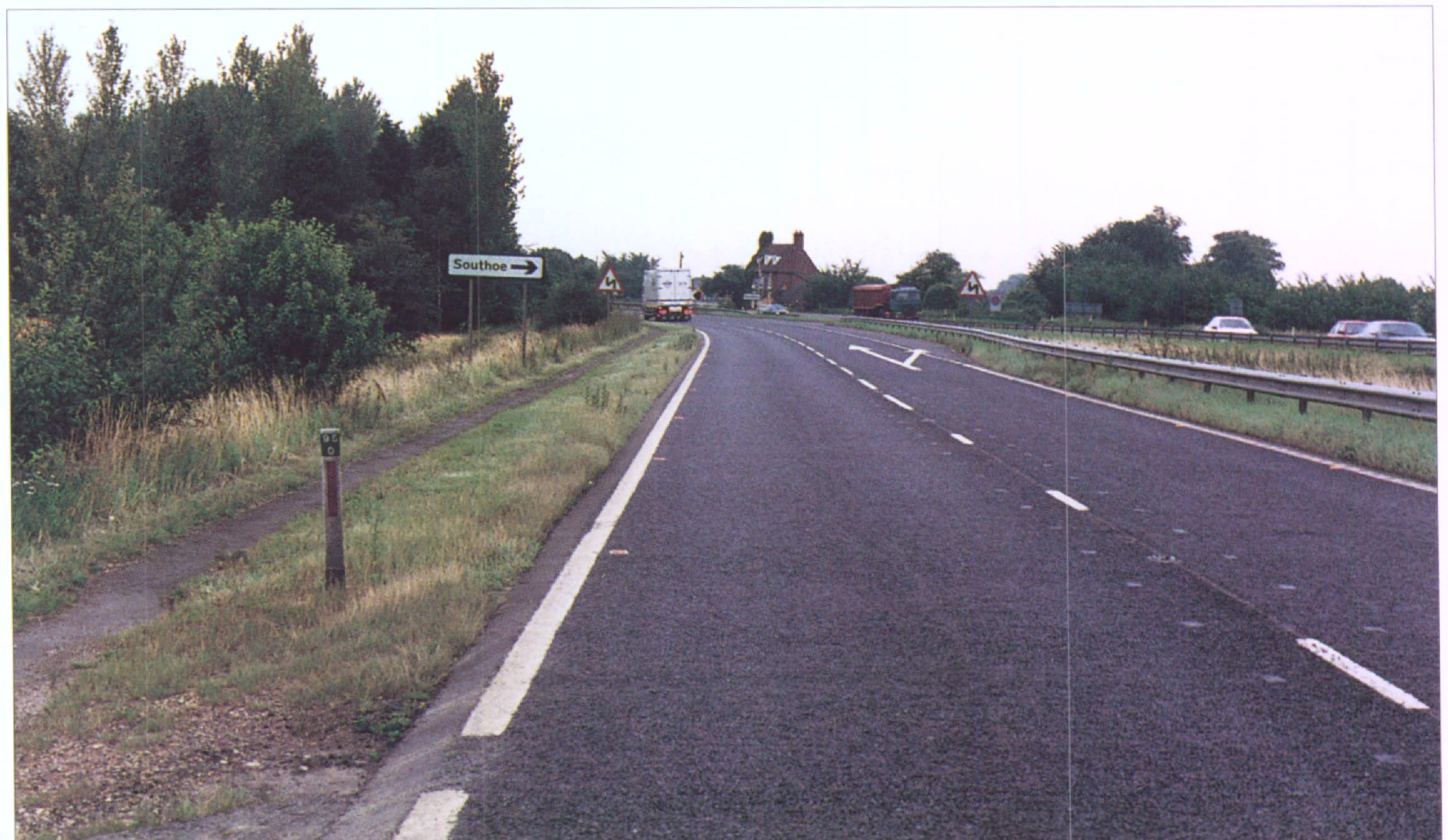
Figure 2.2E Poor forward visibility
