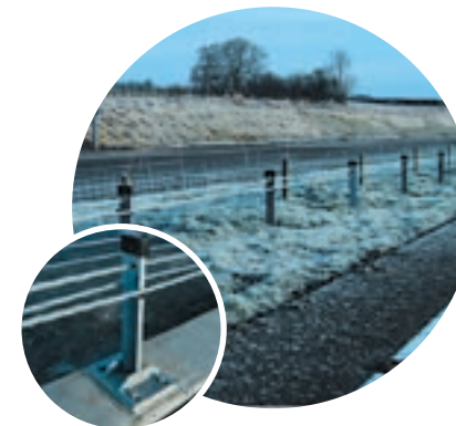
Wire rope safety fence used here on a dual carriageway can also be used as a median barrier on some single carriageways
