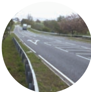
Crash protection is an essential element of road design
